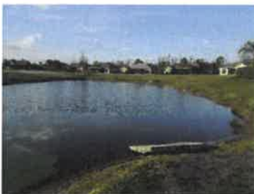
Inflow pipe end section #1 (2018)
