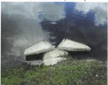
End section on East pond (2018)
