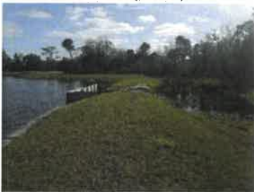
Weir, Skimmer and spreader swale (2018)
