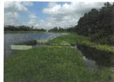
Weir and skimmer (09/2017)
