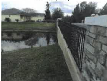
Bridge connection between Pond 7 and Pond 6 (2018)
