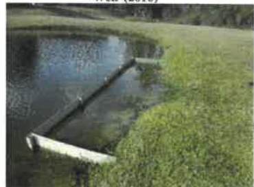
Weir and skimmer (2018)
