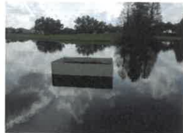
Control Structure after inspection (09/2017)
