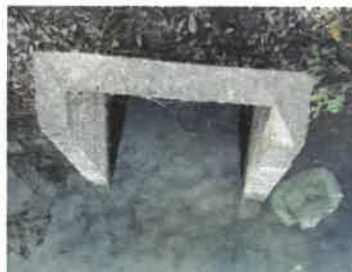
Orifice on south corner of pond (2018)
