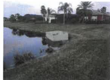
Shoreline and Control Structure (2018)
