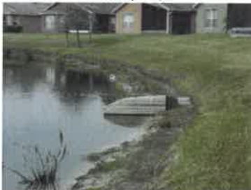
Inflow pipe above water (2018)
