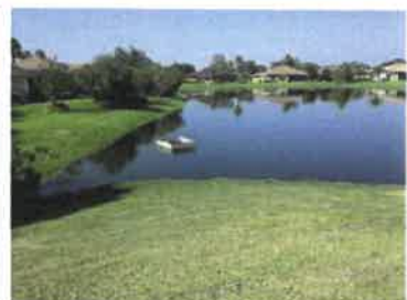
Overall and Control Structure (09/2017)
