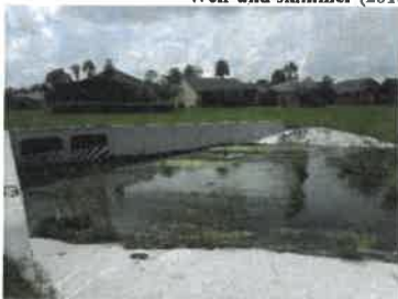
Weir and outflow culverts (09/2017)
