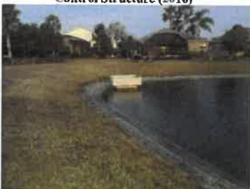
Shoreline and Control Structure (2018)
