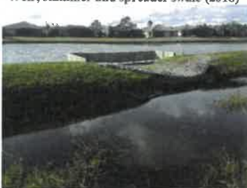
Weir, skimmer and spreader swale (2018)
