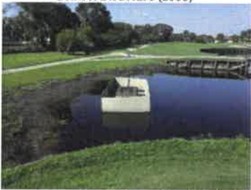
Control Structure and shoreline (09/2017)
