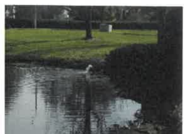
Inflow pipe from pump located at the tunnel (2018)
