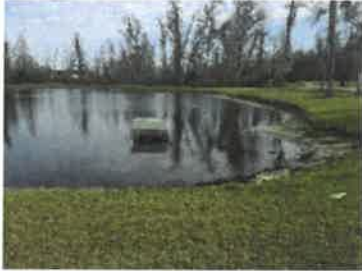
Shoreline and Control Structure (2018)
