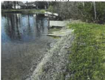
Shoreline, orifice, skimmer and weir (2018)
