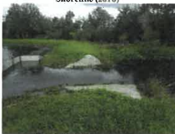
Weir full of water (09/2017)
