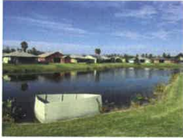
Overall and Control Structure (2016)
