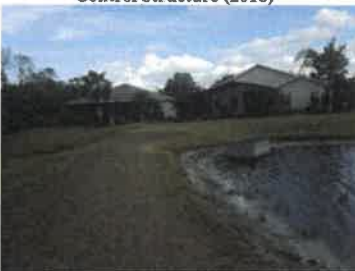
Shoreline and Control Structure (2018)
