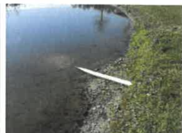
Inflow pipe above water (2018)
