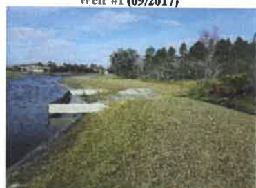
Weir #1, skimmer and spreader swale (2018)
