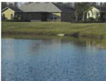
Inflow pipe end section #2 (2018)
