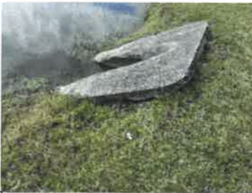
Inflow pipe end section #1 (2018)
