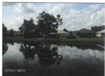
Control Structure under water (09/2017)
