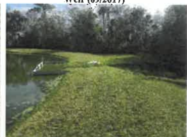
Weir, skimmer and spreader swale (2018)
