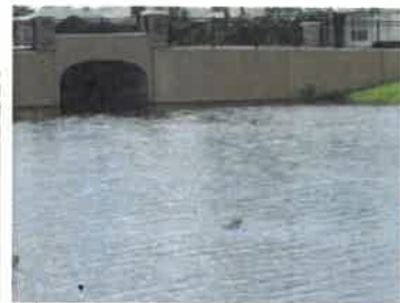
Pond D-9 looking at bridge between Pond D-9 and D-8 (09/2017)
