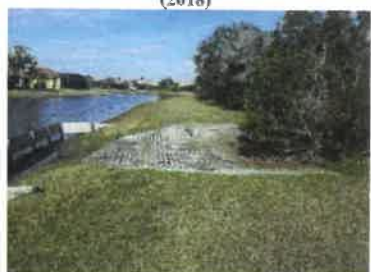
Weir #2, skimmer and spreader swale (2018)
