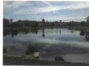
Pond overview and inflow pipe (2018)
