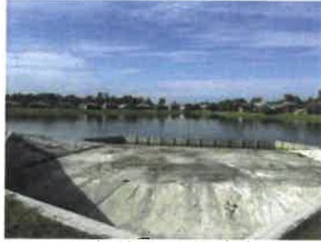
Weir and skimmer (2016)
