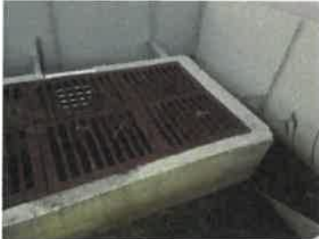
Control Structure Grate (2018)
