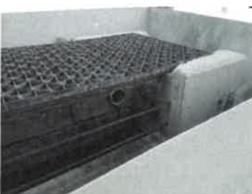
Control Structure Grate (2018)
