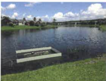
Control Structure at time of inspection (09/2017)
