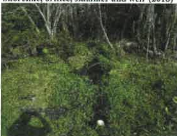
Orifice outflow pipe (2018)
