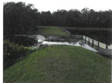
Weir, Skimmer and spreader swale (2016)
