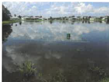
Control Structure under water (09/14/2017)
