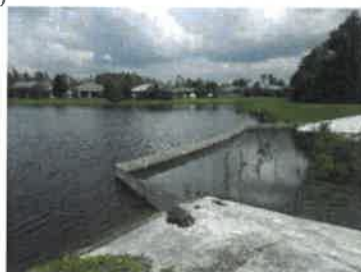
Weir and skimmer (09/2017)
