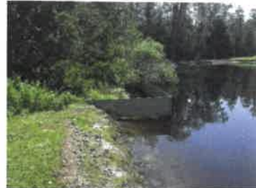
Weir and skimmer (09/2017)
