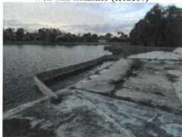
Weir and skimmer (2018)
