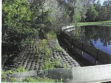
Weir and skimmer (2016)
