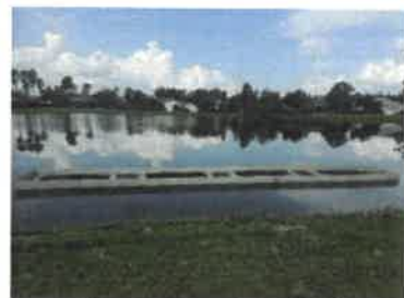
Control Structure at water level (09/2017)
