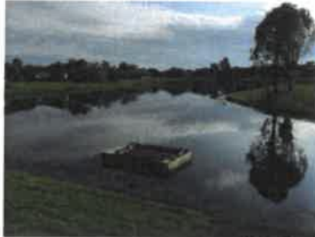
Control Structure and Overall (2016)
