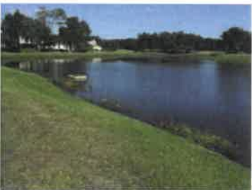
Control Structure and Vegetation (2016)
