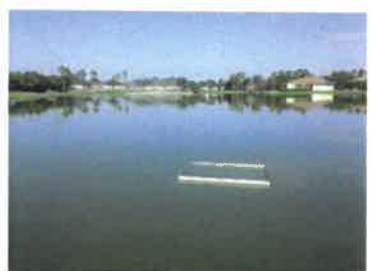
Overall and Control Structure (09/2017)
