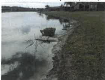
Inflow pipe at water level (2018)
