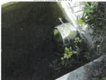
Orifice cleared of debris (2018)
