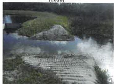
Weir and Spreader swale under water (2018)
