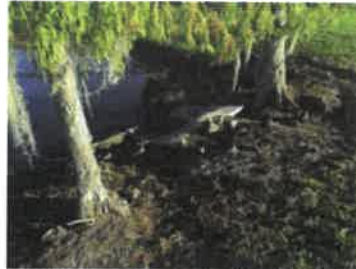
Pipe connecting to Pond E-21(2016)
