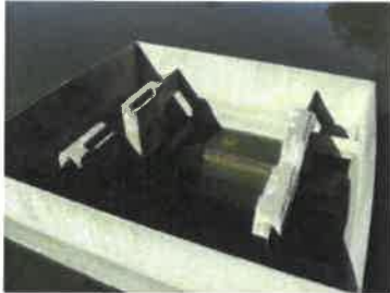
Control Structure and Orifice (2016)
