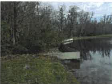
Weir and skimmer (2018)
