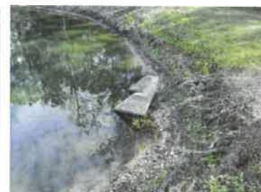
Orifice on south corner of pond (2018)
