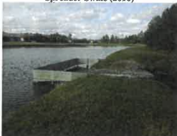
Weir, skimmer and spreader swale (2018)
