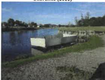
Shoreline and Control Structure (2018)
