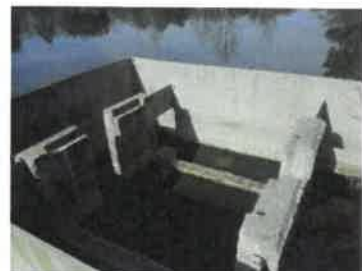
Control Structure and Orifice (2018)
