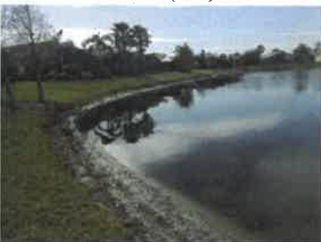
Shoreline and inflow pipe end section (2018)
