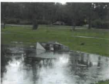
Control Structure after inspection (09/2017)
