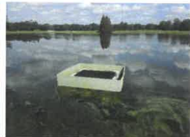
Control Structure after inspection (09/2017)
