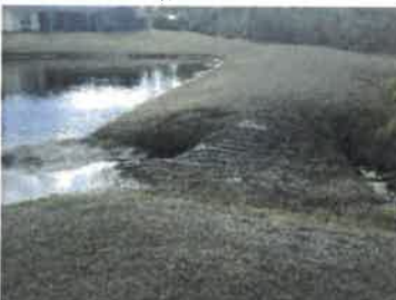
Weir and spreader swale (2018)
