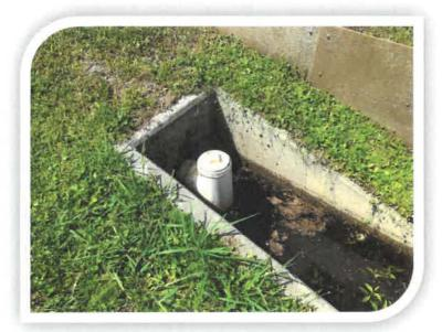
Missing 6" tees and caps were added to drain orifices as needed.
