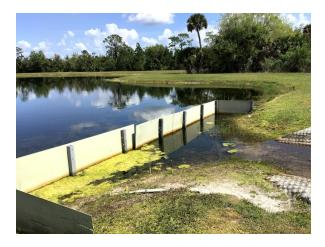
Pond D-4 Minor Erosion around weir.
