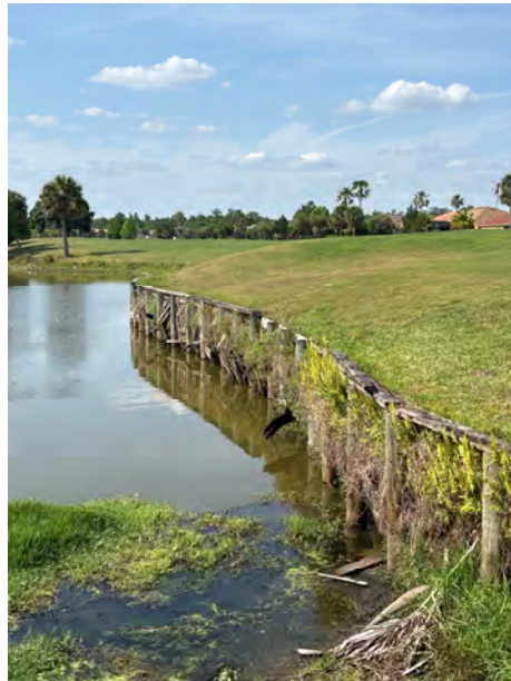
Retainig walls deterioration and debris accumulation is observed.
