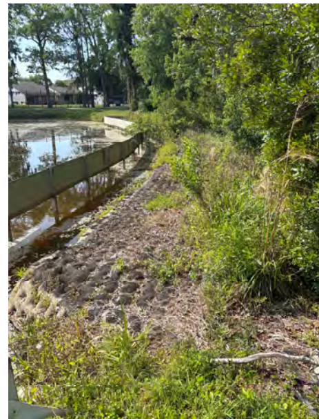
Spillway, Weir, and skimmer are in good condition However overflow weir is covered by vegetation.
