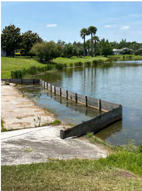
Weir and skimmer appears to be working properly.
