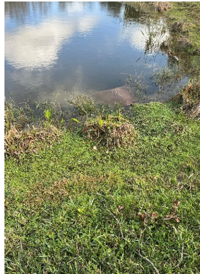
Submerged concrete pipe appears in good condition and functions properly.
