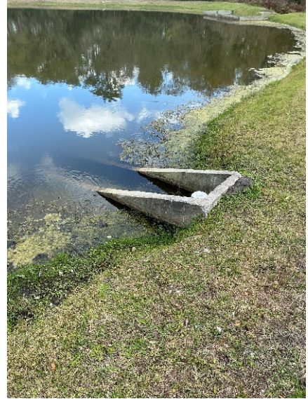
MES appears in good working order. Algae surrounding structure.
