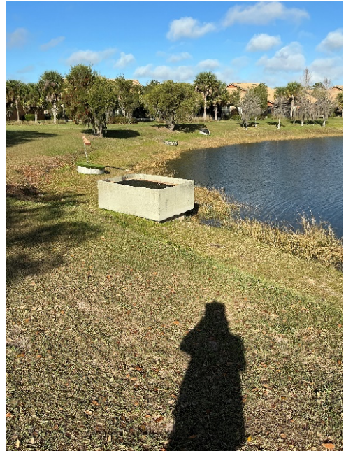
Control structure appears in good working order.
