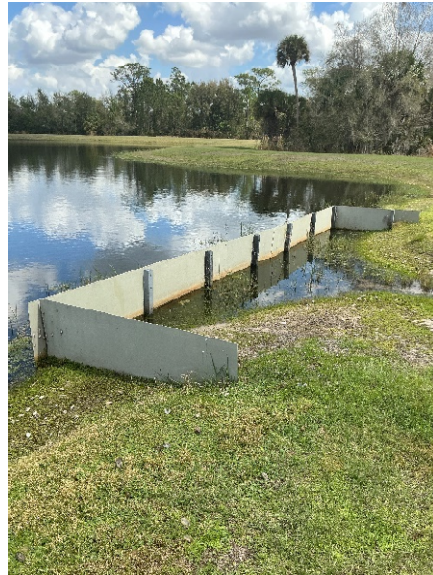
Weir/spillway appears to function properly.
