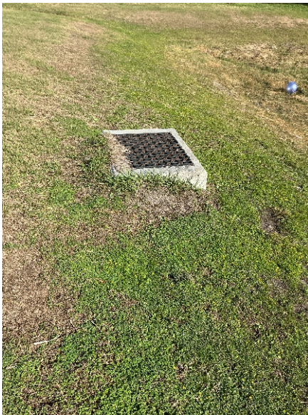
Control structure appears in good working order. Slight debris overtop.
