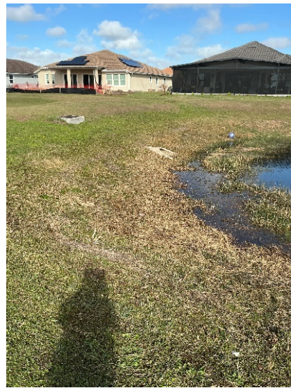
RCP pipe appears undamaged and in good working order.
