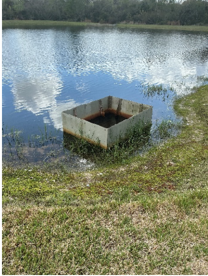
Control structure appears in good working order.
