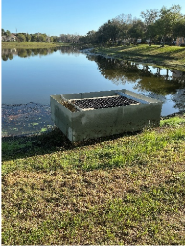
Control structure appears in good working order.
