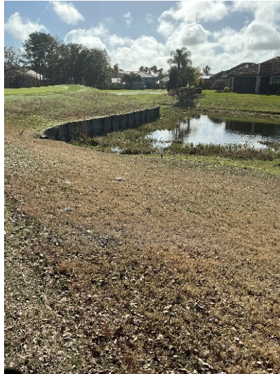
Retaining wall appears to be in good shape.
