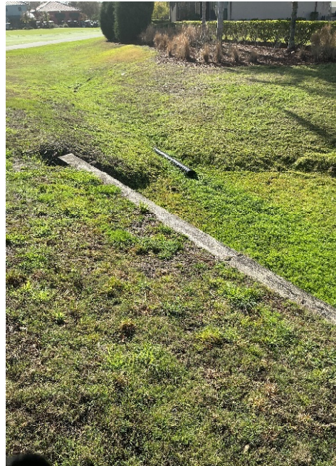
Corrugated pipes appear undamaged and functioning properly.
