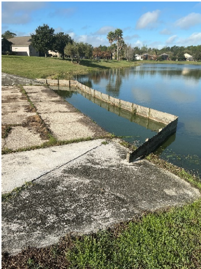
Weir/spillway appears in good working order.
