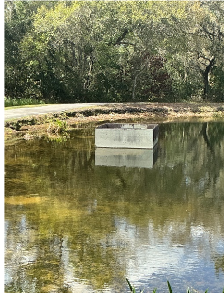
Control structure appears to be in good order.
