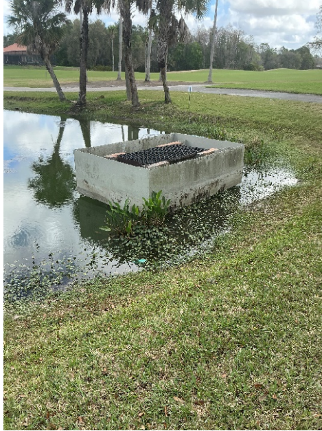
Control structure appears in good working order.
