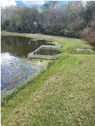
Weir/spillway appear to be functioning properly.
