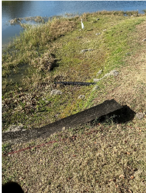
Corrugated pipes appear undamaged and functioning properly.
