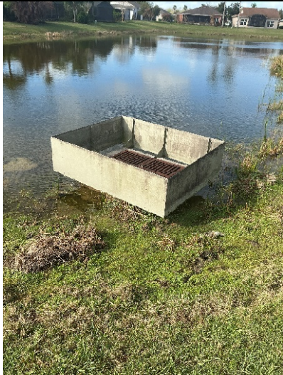
Control structure appears in good working order.
